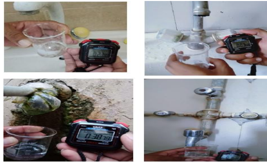
Fig.2 Measurement of leaks at various places
